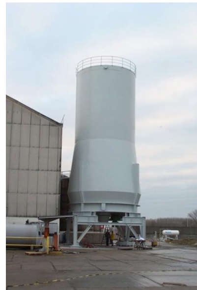
Rotor 8.000; 150 t/h FGD-Gypsum incl. Silo
