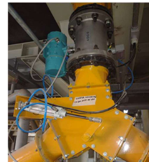
Two of the three installed DYNAmas (DN80), Pneuma. Conveying
