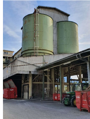
two conveying lines into the silo
