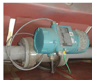
Two of the three installed DYNAmas (DN80), Pneuma. Conveying
